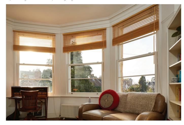
The system has two sashes built into the frame which slide in opposing directions and will remain fixed in any position.
